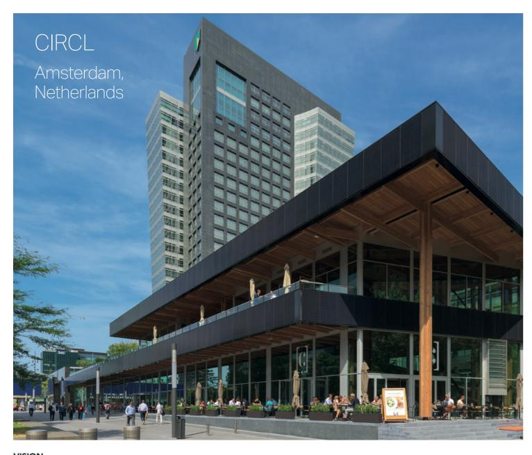
A new pavilion in Amsterdam's Zuidas district, CIRCL was designed and constructed according to sustainable and circular principles. Energy efficient and easy to disassemble, many of the raw materials are recycled and can be put to different uses in the future, including the aluminium envelope.
