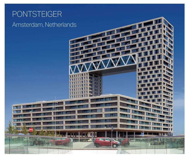
Pontsteiger is an integral part of transforming the former lumber port of Houthaven into an aspirational neighbourhood. This spectacular residential building is an incredibly complex project, involving a 'bridge' constructed with four steel lattice trusses hung between two 90m high towers, emanating from the IJ river.
